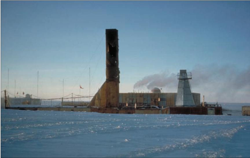
Fig. 1: Drill units at the Russian Vostok Station in East Antarctica.
