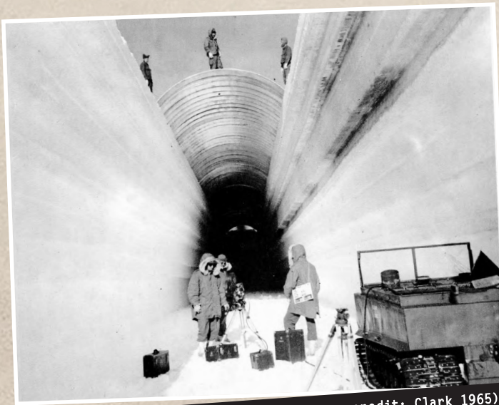
Figure 6: Roofing a finished trench (image credit: Clark 1965).
