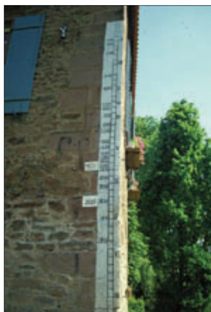
Fig. 1: Flood marks at Wertheim on the tributary of the Tauber river to the Main (Glaser, 2001)
